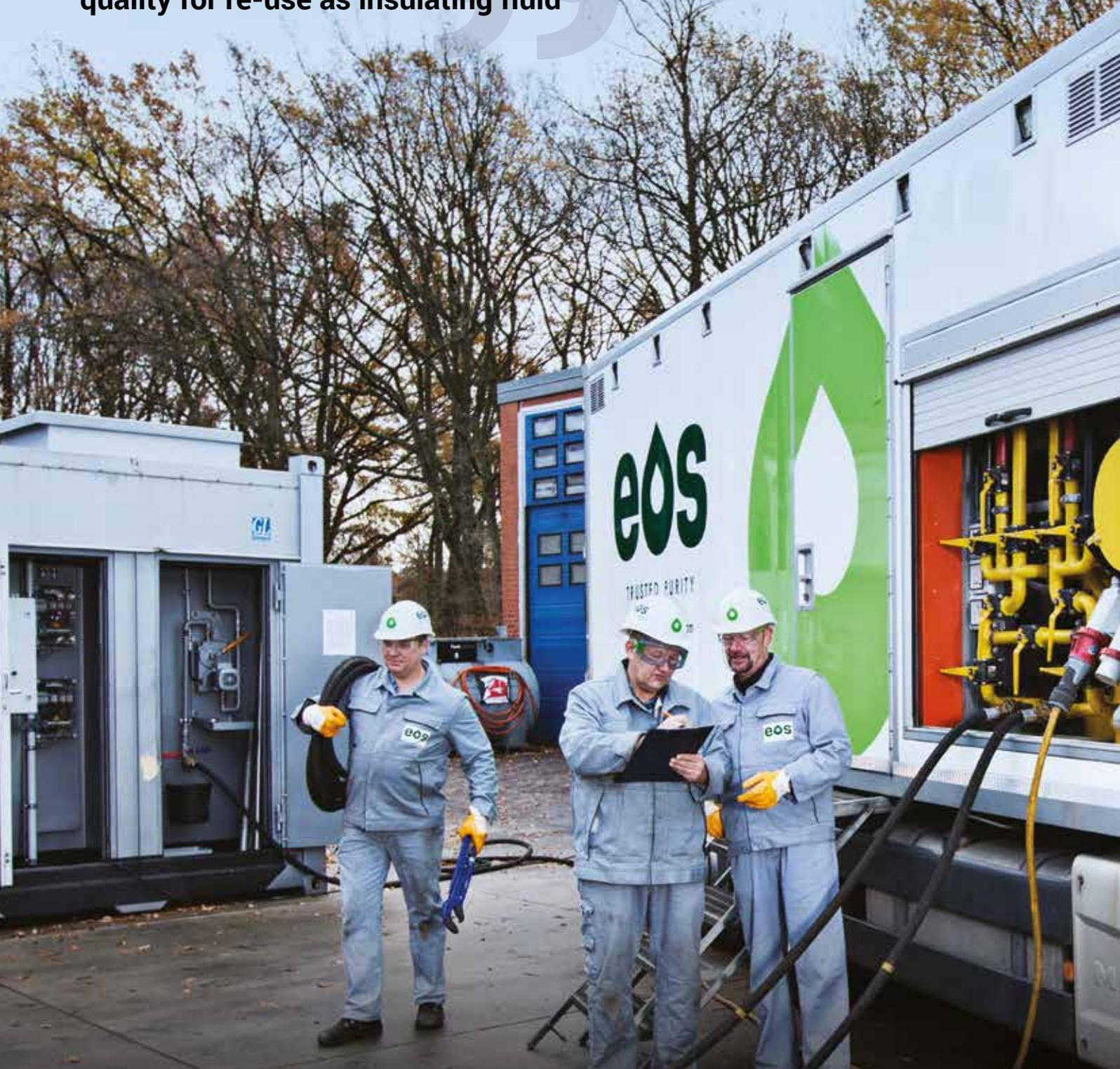
Used transformer oil (UTO) is a valuable resource because it can be processed to “as new” quality for re-use as insulating fluid. Customers in the electricity transmission and distribution
